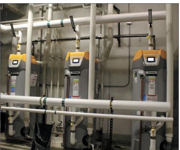
The old hot water heaters which heat different areas of the school were recently replaced with improved ones. "The new HVAC system requires additional hot water heaters and the existing hot water heaters were old and needed to be replaced," Rippe said. Photo by McKenzie Gandy
